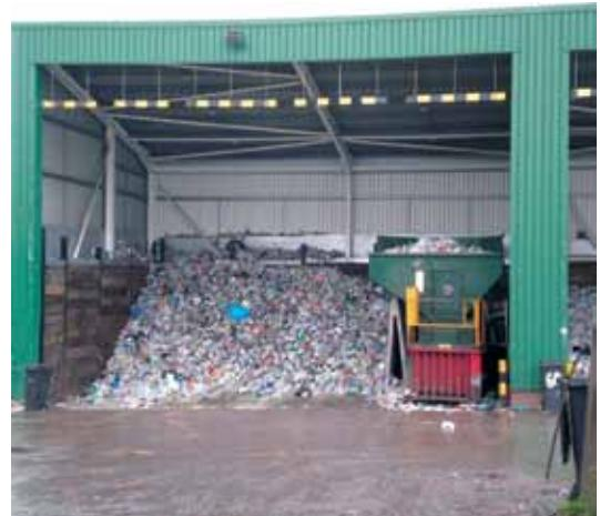
Figure 5 Illustrative photos of a Municipal Waste Transfer station (Storage discharge type)
